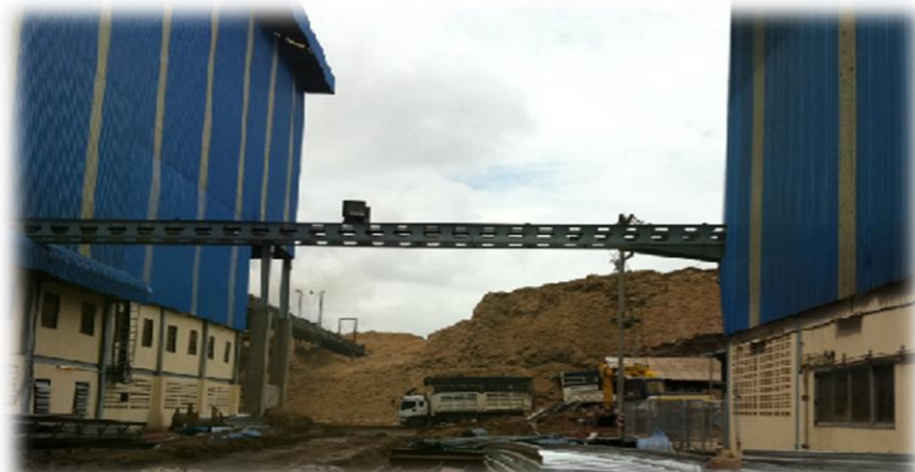
Erawan Power(Sugar cane power plant )
