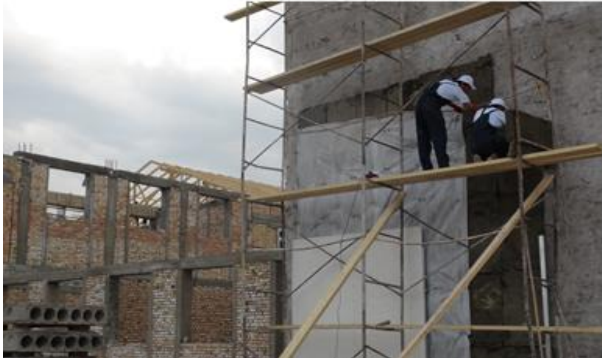
External insulation of walls of new buildings in Kyrgyzstan
