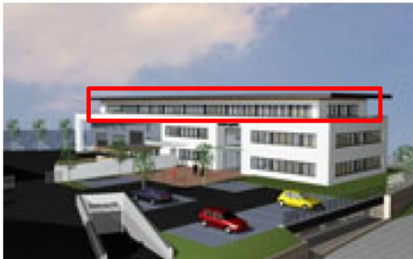
Service building St. Johann with critical room
