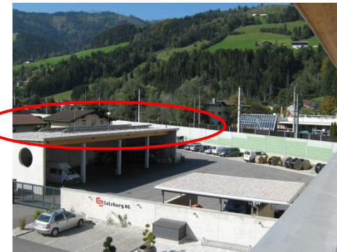
PV system 5 kWp
