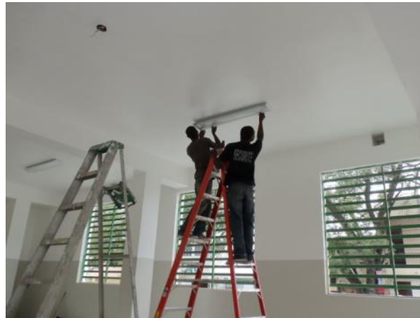
Installation of ceiling lamps, outlets and fans
