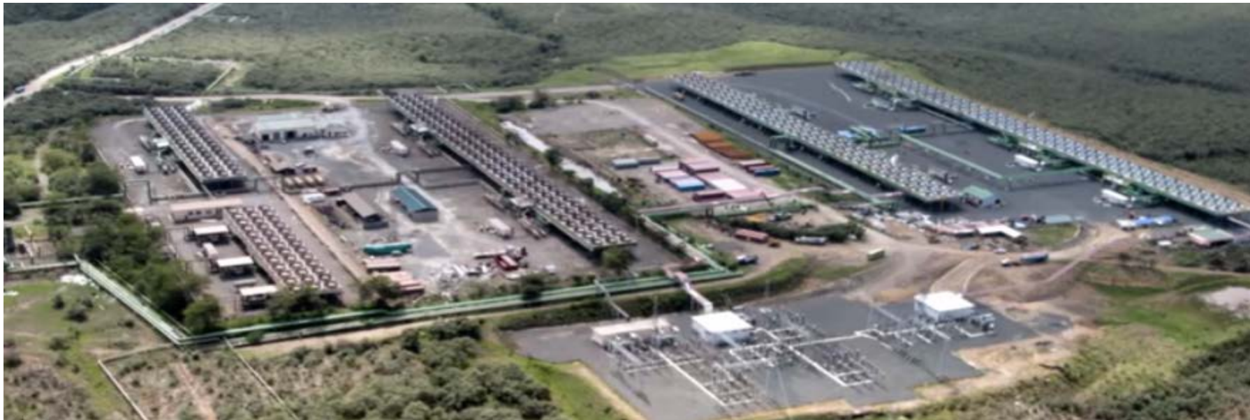
Olkaria III Geothermal Plant in Kenya by Ormat (source: ThinkGeoEnergy)
