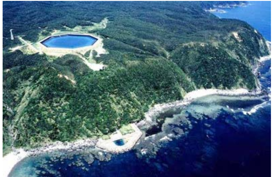
Yanbaru Plant seawater pumped hydro storage in Okinawa, Japan
