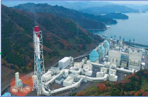
Coal fired plant with solid sorbent for CO2 capture
