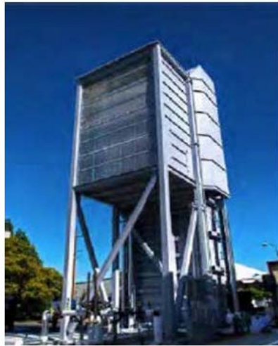
Initial Pilot Plant GT DAC 1
