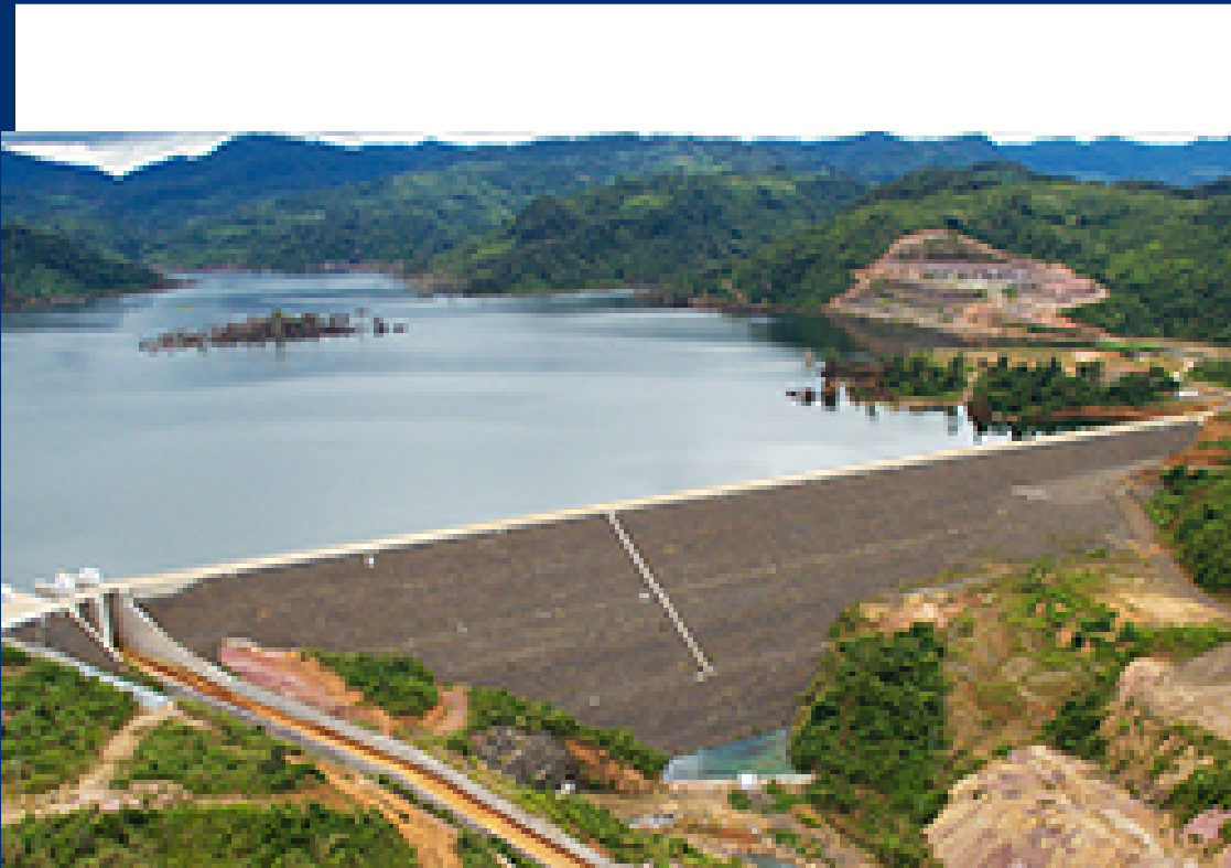
Figure. Houay Lamphan Gnai Hydropower plant, Champassak province
