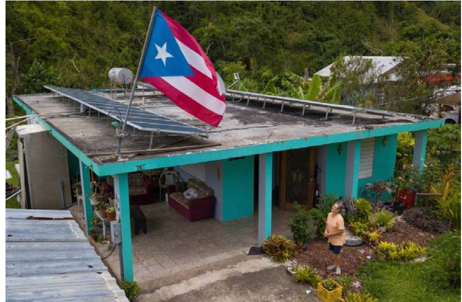
A part of a micro-grid solar power project in Puerto Rico
