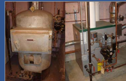
3. Heating System Repl.
